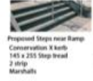
Proposed Steps near Ramp Conversation X kerb 140 x 255 Step tread 2 100p Marshalls
